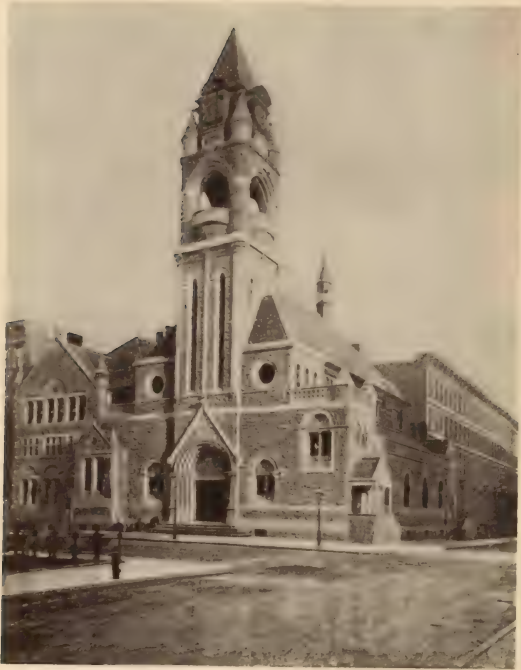
MADISON AVENUE M. E. CHURCH 60th Street and Madison Avenue. R. H. Robertson, Architect. (1884.)
